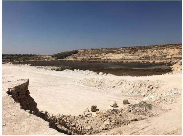
Photo 2: Wastewater Pond 3B, Sep. 2019
